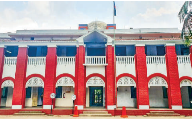
Dr. M. A. Rashid Administrative Building
