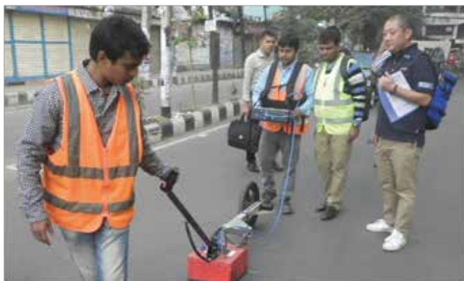
Ground Penetration Test is being performed to Scan Underground Utility Lines
