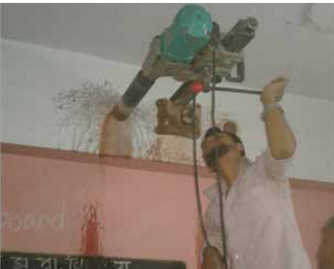
Core Cutting is being performed
