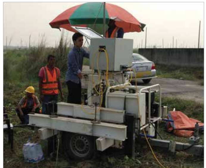
Cone Penetration Test is being performed
