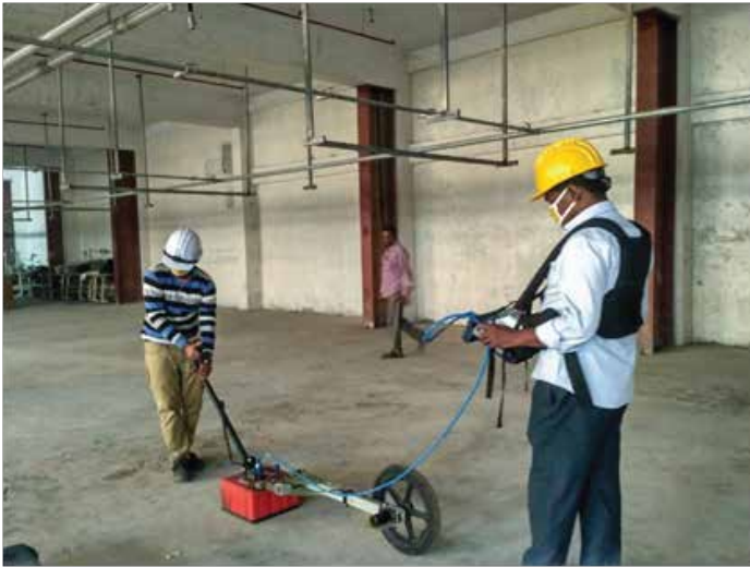
GPR Survey is being conducted at HR Textile Mills Ltd., Savar, Dhaka
