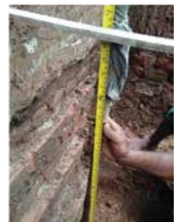
Checking the Foundation during Seismic Vulnerability Assessment
