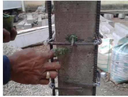
Figure 2: Application of Epoxy Chemical
