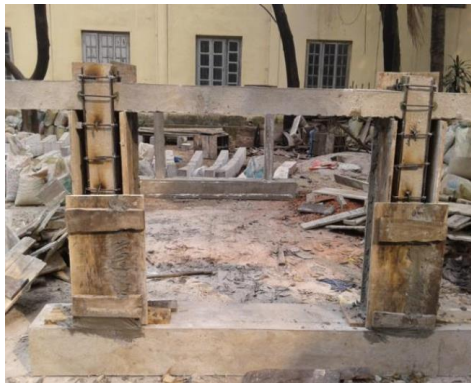
Figure 3. Formwork for a widening of column
