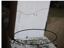
Figure 17. Crack Pattern at Beam-Column Joint
