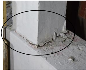
Figure 24. Crack Pattern at Column-Base beam Joint
