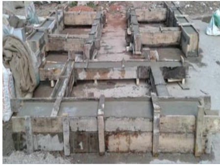
Figure 1: Horizontal Concrete Casting
