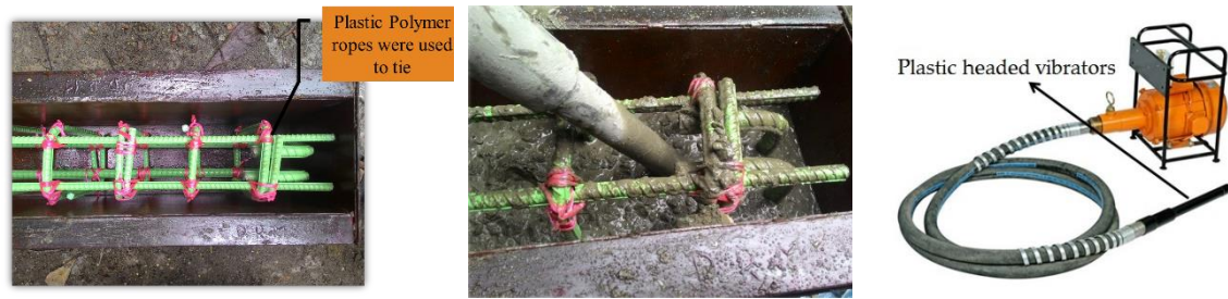
Figure 3. Precautions taken during concreting.
