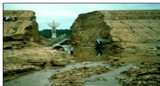
Figure 2. Failure of embankment constructed on dispersive soil (Missipi, USA)
