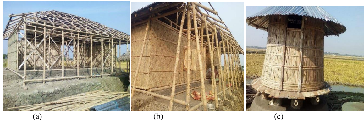
Figure 4. Implementation of design. (a) Structural frame of the house. (b) Structural buttresses to provide extra protection of the main structural system against strong and lateral forces. (c) Granary for food security.
