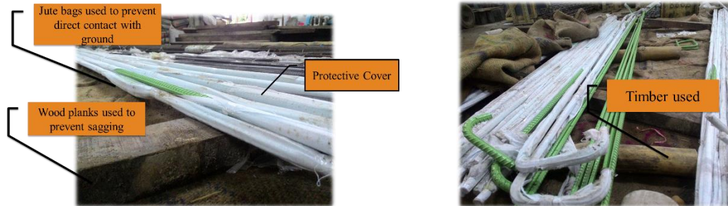
Figure 1. Precautions taken during storage of coated bar
