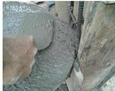
Figure 4. Micro-concrete placement
