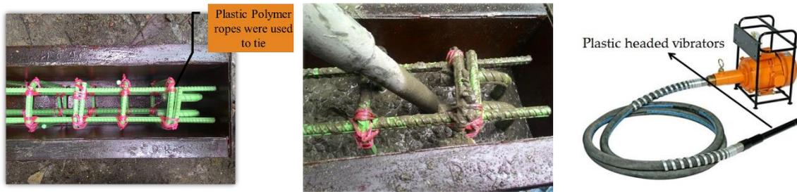
Figure 3. Precautions taken during concreting.
