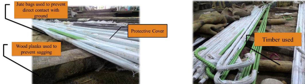
*Figure 1. Precautions taken during storage of coated bar*
